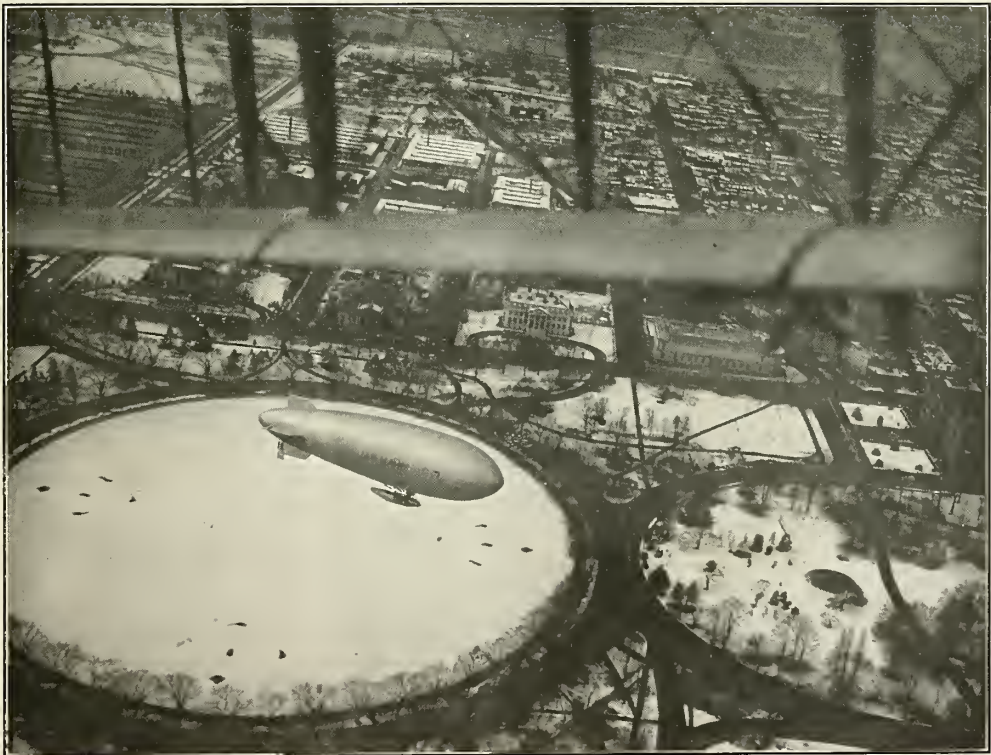
The first helium filled airship in the world, the Navy Blimp C-7 over "ellipse" at Washington
